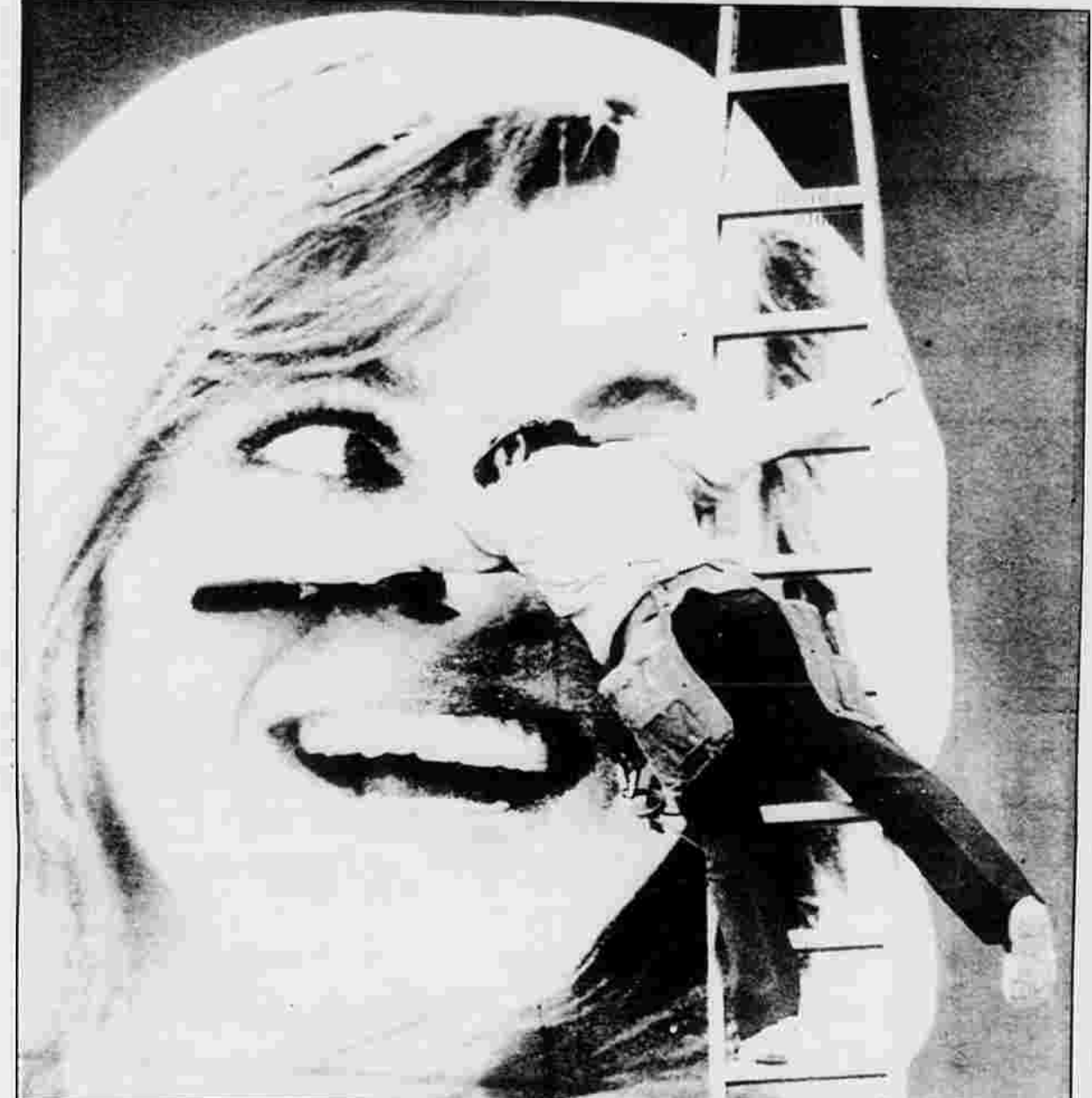
REPAIRS — Dennis Doyle pastes down pieces of an outdoor billboard in Austin, Texas, Tuesday. Doyle said it takes about an hour to replace the entire board, which is done every two months as the message fades.
